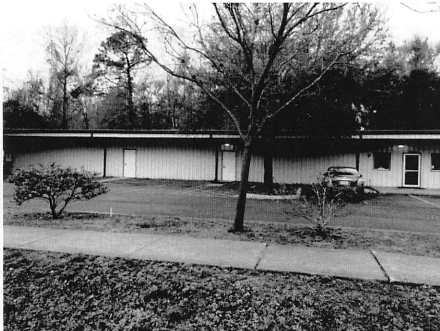
Warehouse/office structure across Dahlia Street from the subject site
